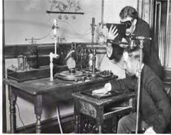
Thomas Edison is seen viewing the hand of his unfortunate assistant, Clarence Dally, through a fluoroscope of his own design. Dally's hand rests on the box that contains the x-ray tube.
